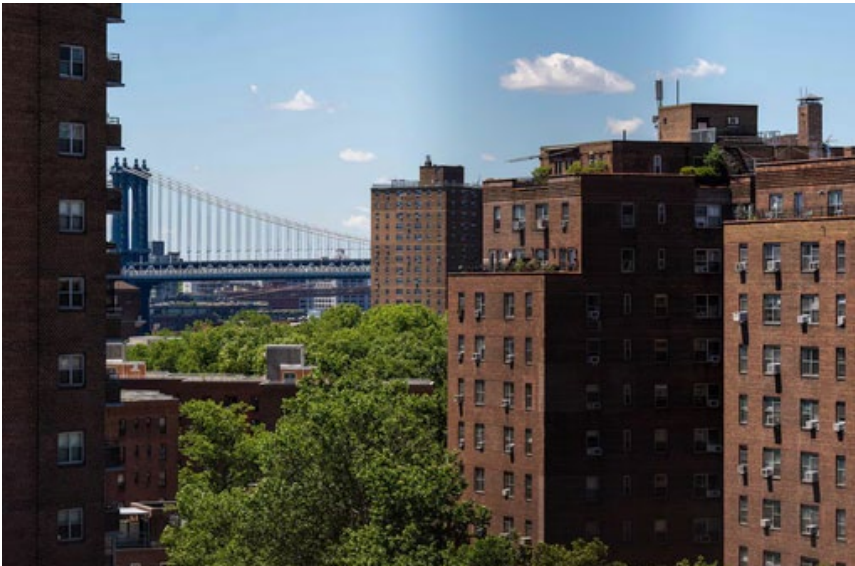
Residential apartment buildings in New York City
